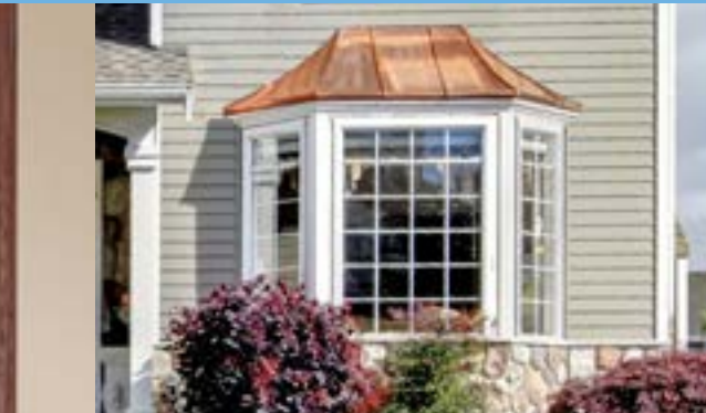
45° Bay with Copper Clad Roof
