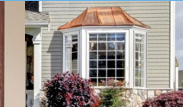
45° Bay with Copper Clad Roof
